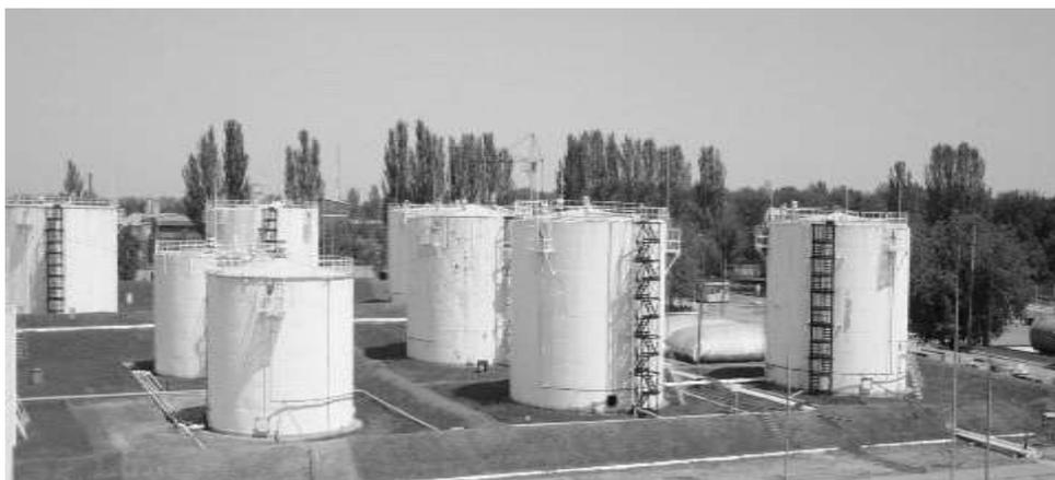
Figure 1 – Oil tanks type RVS (RVS-5000, RVS-3000)
